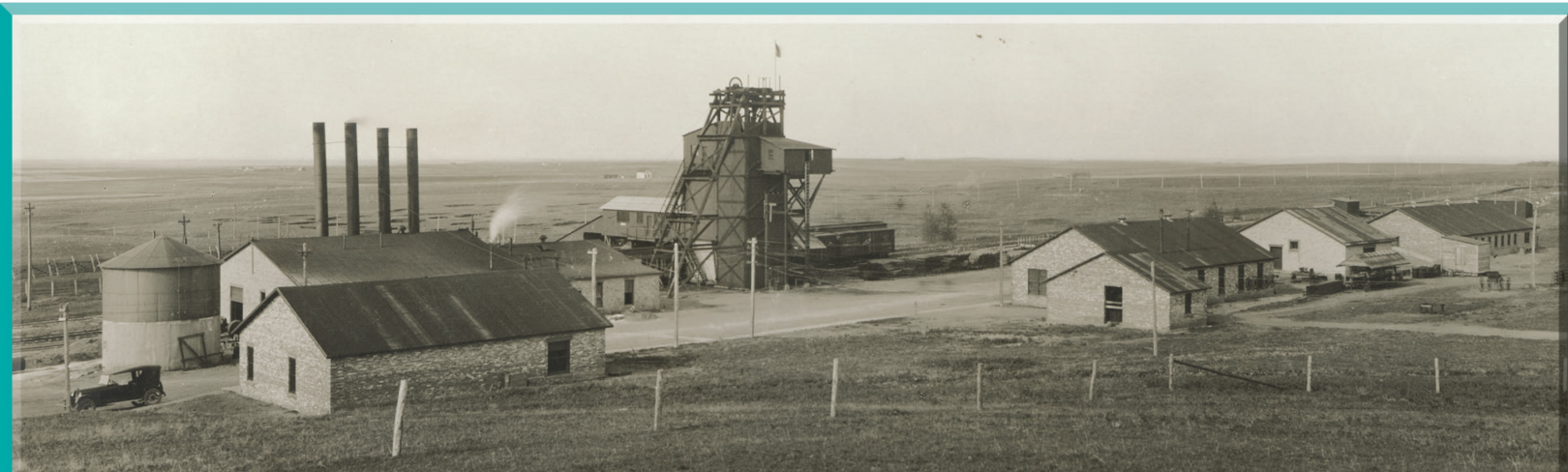
Figure 5. This photo shows the brick buildings and tippel of mine #2 at the Washburn Lignite Coal Company, probably about 1919. Notice the coal cars at the far right. (SHSND 0410-117)
