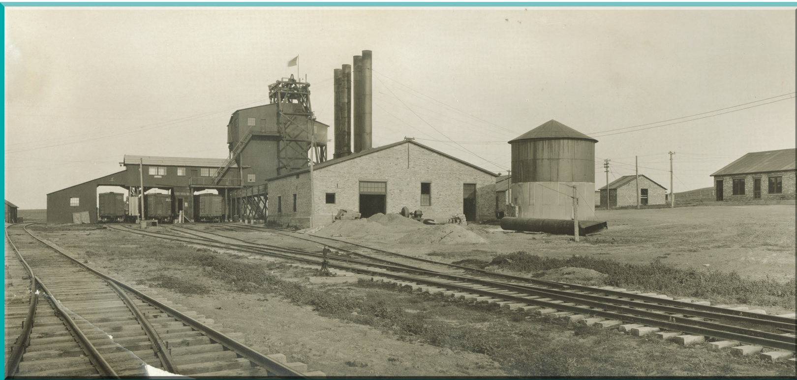
Figure 11. This view of the WLCC tipple shows railroad cars being filled with coal. (SHSND 0410-098-2)
