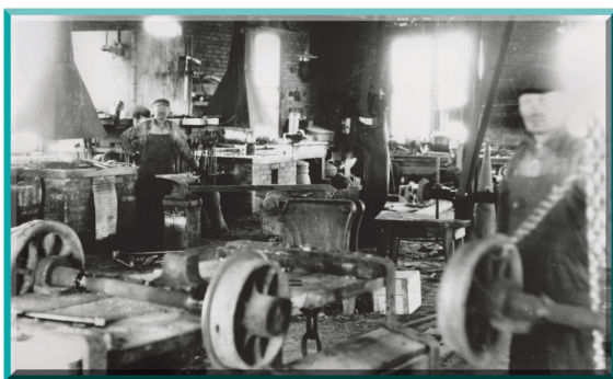
Figure 9. The machine shop at WLCC mine #2. Note the car wheels being repaired. (SHSND A2776)
