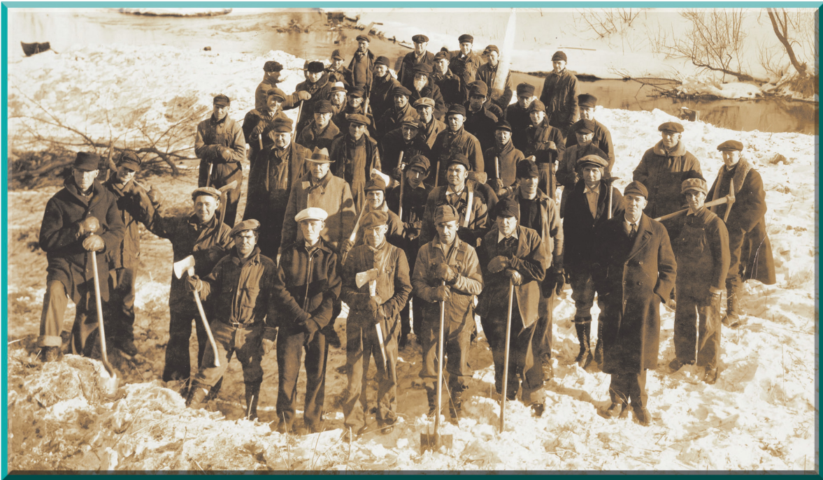
Figure 14. A Works Progress Administration (WPA) work crew on a river cleanup project in Fargo, about 1936. (Institute for Regional Studies, NDSU, Fargo, 2065.35.1)
