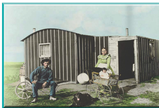
Figure 1. An unidentified family in front of a small tar paper-covered house, with an arched roof. (Fred Hultstrand History in Pictures Collection, Institute for Regional Studies, NDSU, Fargo, 2028.119. Photo by Job V. Harrison of Rock Lake, ND)
