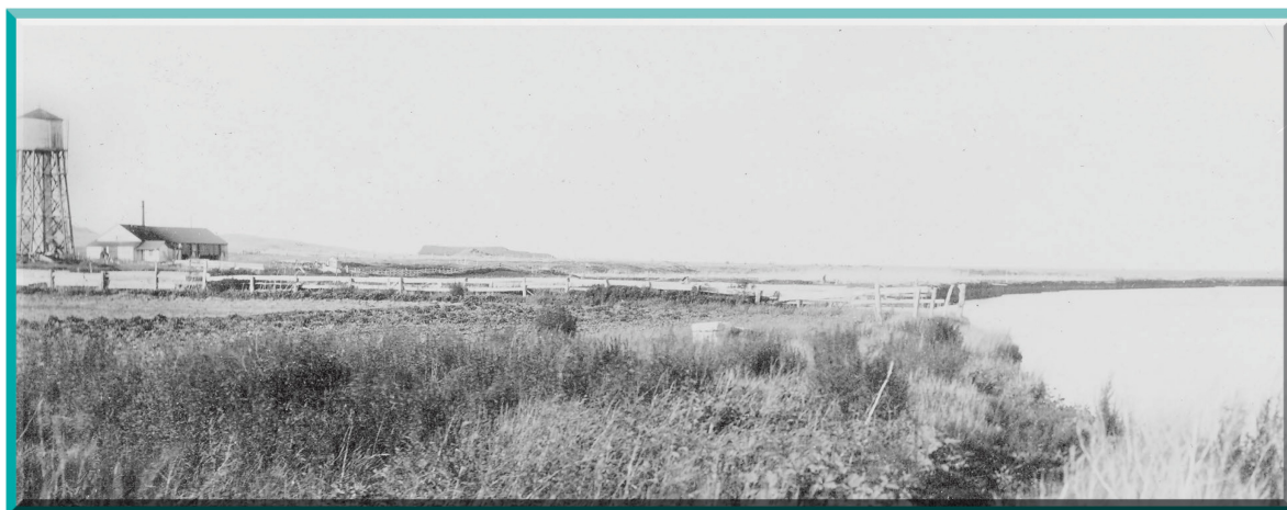
Figure 3. Fort Buford water tower and sawmill, 1891–93. Post surgeons reported diseases such as diarrhea, dysentery, and typhoid fever that we know today result from contamination of drinking water by human and animal wastes. In the 1880s the post began drawing its drinking water from the river instead of from wells, and such illnesses were reduced. In the 1890s waterworks replaced drawing water directly from the river. (SHSND C0765)
