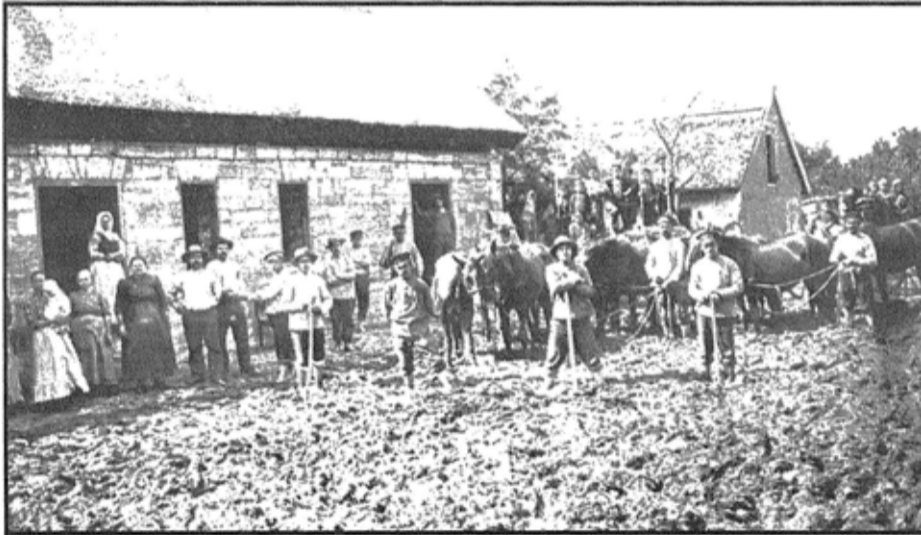
Here, Germans living in Russia are mixing clay and straw to make bricks. When some of the Germans from Russia came to North Dakota, they built houses and even churches of the same mixture, as shown below in the photograph of a Lutheran Church near Hazen in 1914.
