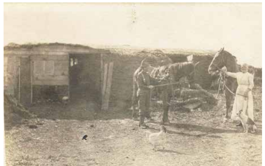
Building homes on the prairie proved a challenge to many settlers, who turned to building their homes by cutting sod to make walls. Many sod homes were half dug out of the ground.
