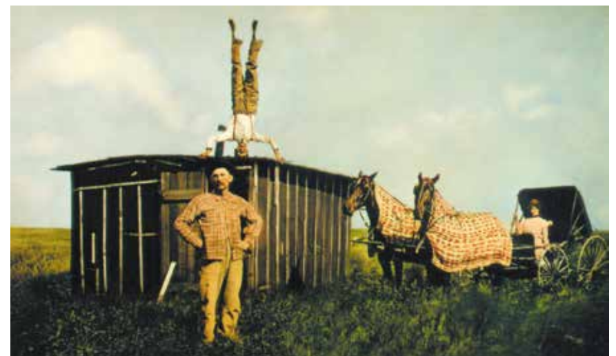
A few years later, as supplies became more accessible to get, settlers constructed their homes by building a lumber frame and then layered tarpaper over it.
