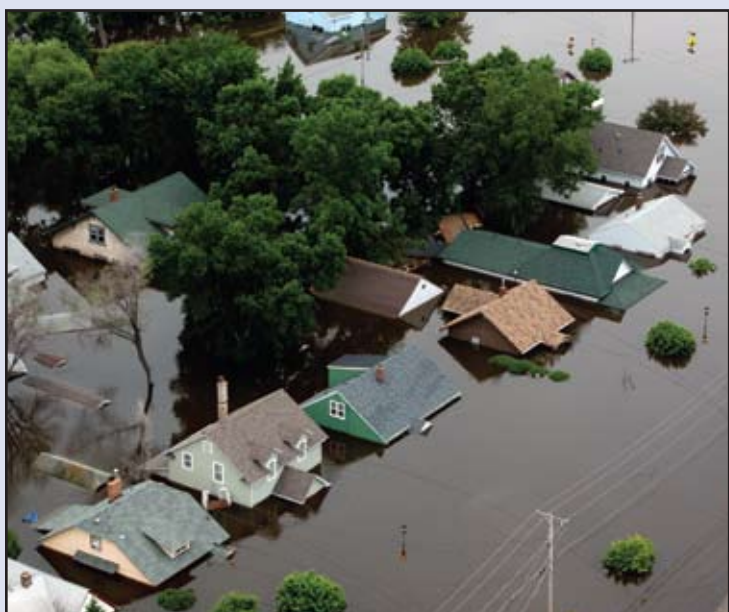
Mouse River, Minot. In June 2011, the Mouse River through Minot reached record levels, resulting in the evacuation of more than 10,000 residents. Approximately 4,100 homes and businesses experienced major flood damage. (FEMA photo)
